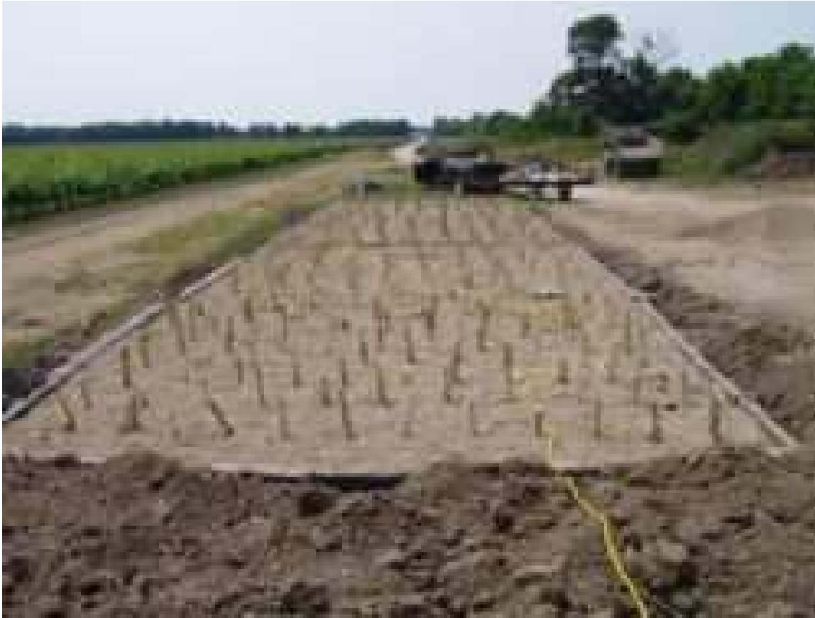
Photo 13.2 Newly Planted Constructed Wetland
